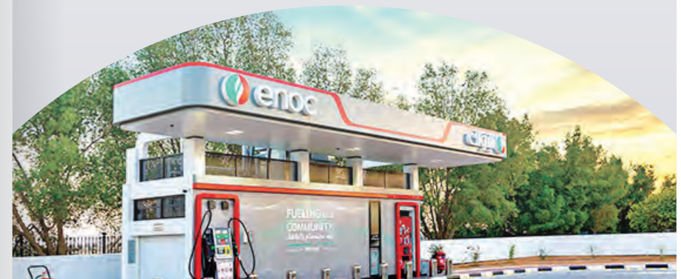
ENOC compact retail station in Dubai
